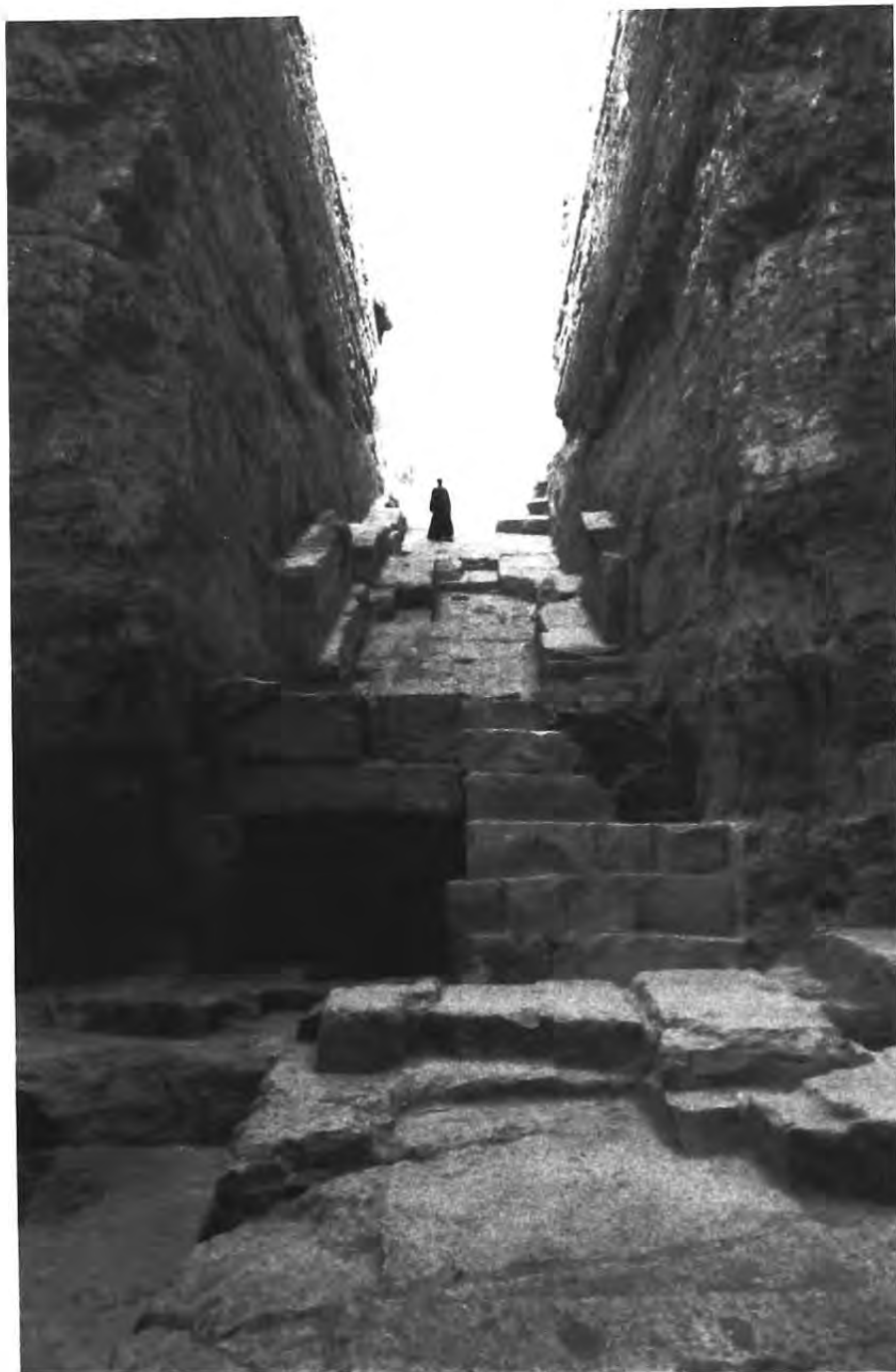
ABU ROWASH. The central section of the foundation level and the cleared descending ramp. (Photograph by M. Vallogia, 1997)
